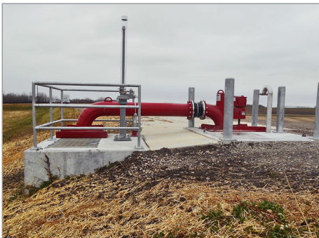
Gatewell D and new pump station
