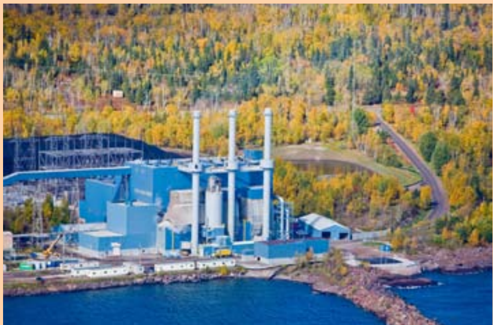
Taconite Harbor Power Plant, Schroeder, Minnesota
