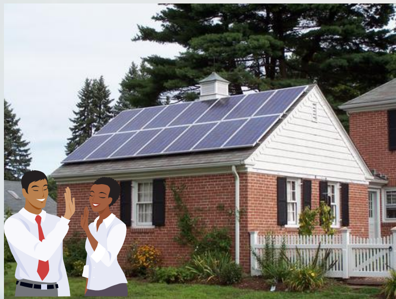
Photo credit: groSolar (NREL PIX)
