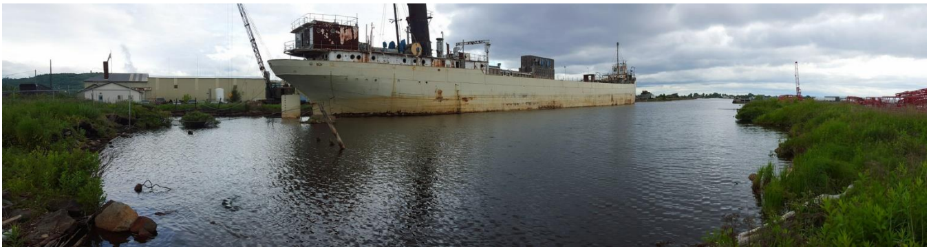
The Azcon Corp/Duluth Seaway Port Authority Garfield site, a 6.4-acre slip used for docking ships, with an operating scrap yard to the north. Contamination includes polycyclic aromatic hydrocarbons, lead, zinc, and dioxins.
