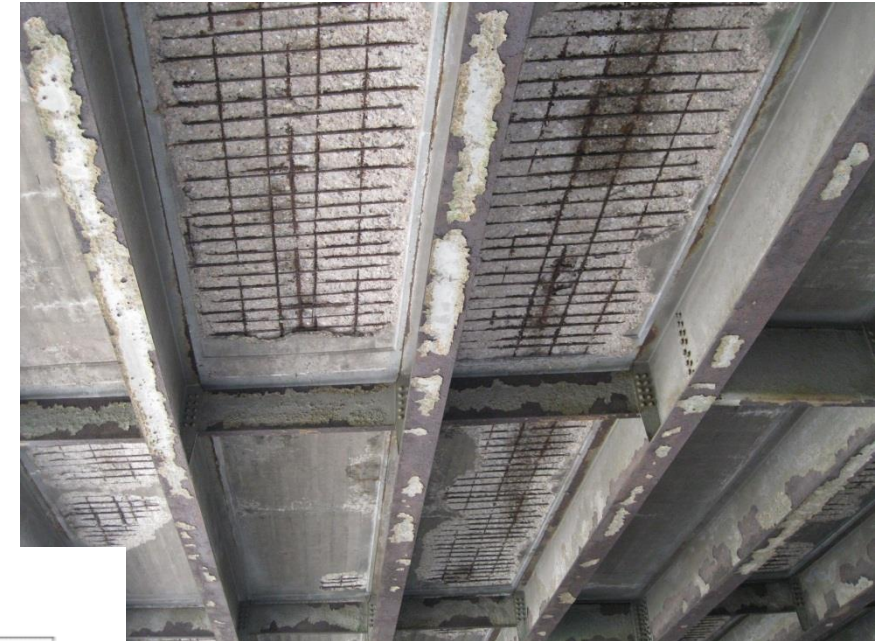
Maryland Ave. over I-35E (before reconstruction)
