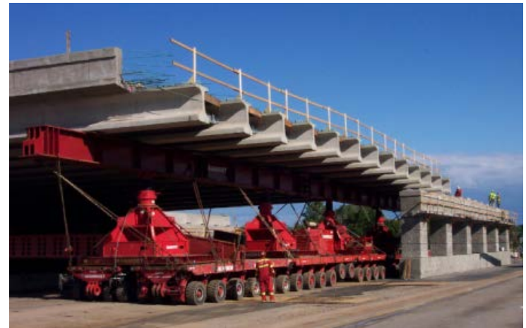
Maryland Ave/I-35E bridge
