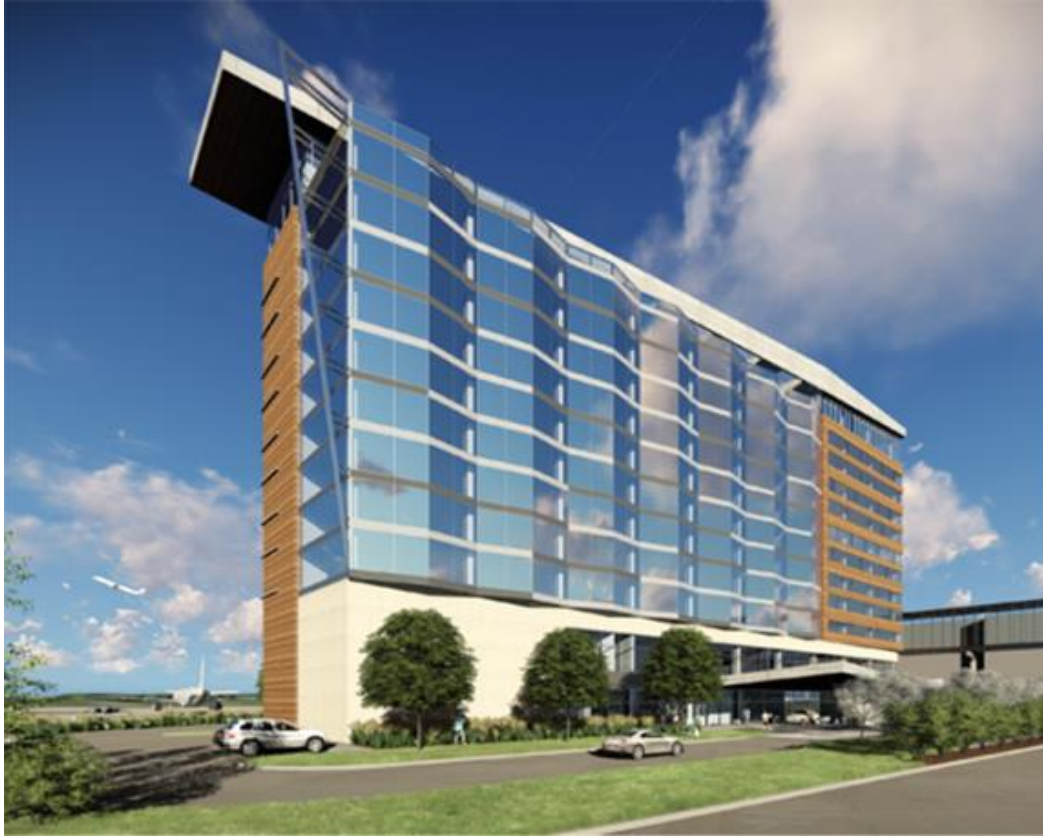
300-room Intercontinental hotel and conference center
