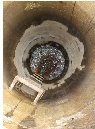
Infiltration at Manhole Structures
