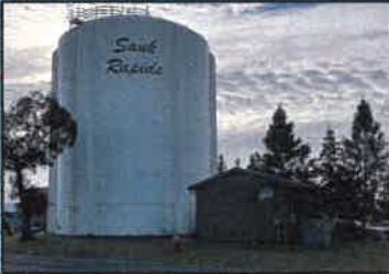
GROUND STORAGE TANK AND BOOSTER STATION
