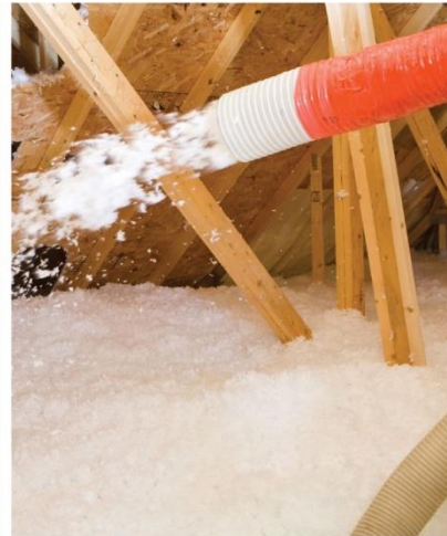
Attic insulation & air sealing
