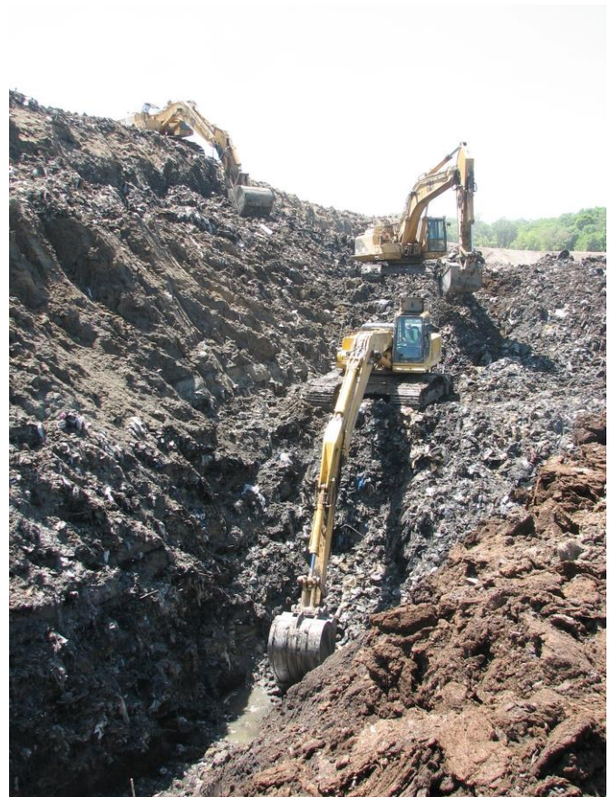
Excavating garbage at a closed Minnesota landfill
