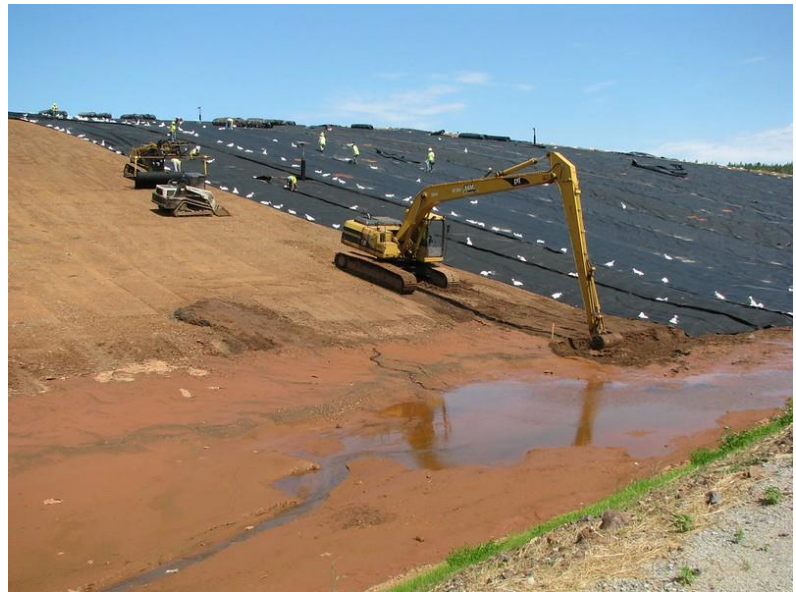
Covers and liners help keep contaminants in landfills from affecting groundwater and other natural resources. The MPCA is requesting authority to negotiate covenants to help protect such measures.
