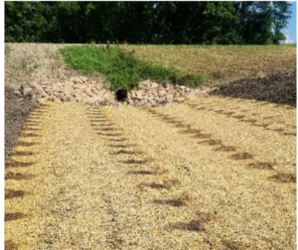
Completed grassed waterway project
