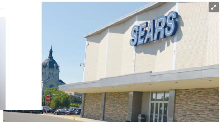
The former Sears store at 425 Rice St. is located near the State Capitol in St. Paul. NANCY KUEHN | MSPBJ
