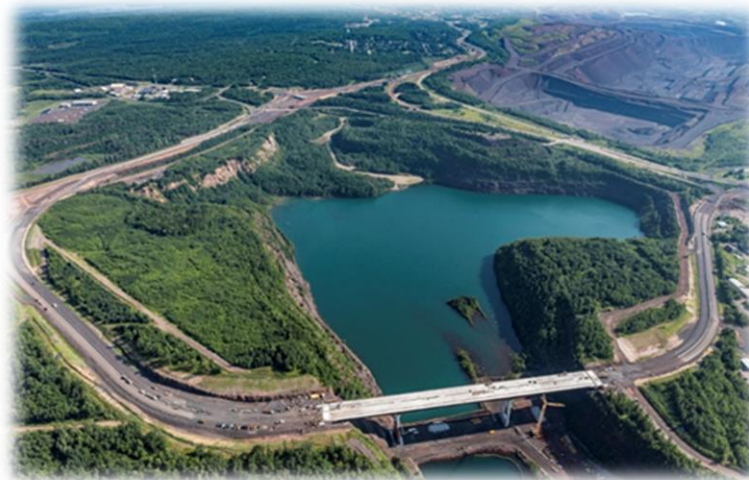
Highway 53 Relocation in Virginia
