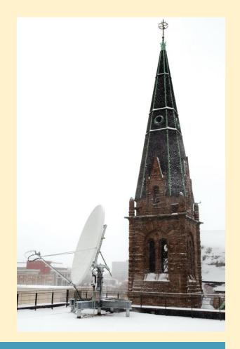
The Uplink Satellite provides the broadcast, Emergency Alert, and AMBER Alert signals to the MPR regional radio network. Photo by Eamon Coyne, MPR Broadcast Engineer.
