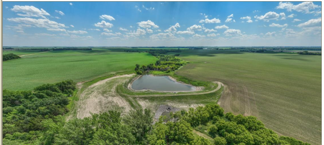
SPRINGDALE 19 GRADE STABILIZATION (Redwood County, 2021)
