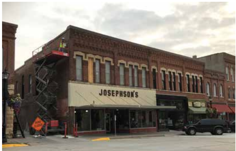
Photo of Red Wing's downtown housing conversion from Red Wing HRA
