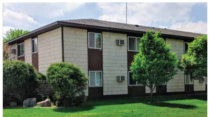
Photo of Gar-Mar Court in Kerkhoven MN
