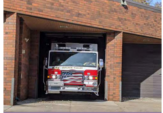
Larger, modern fire equipment is a tight fit in the current buildings.
