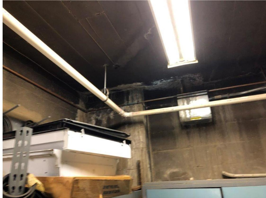
Age, Build-up in Waste Piping, Inadequate Slope for Low Flow Fixtures, Insufficient Valving
