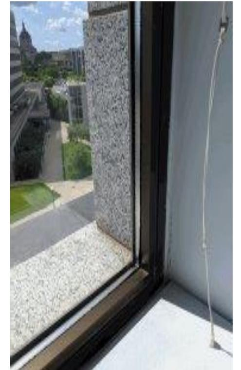
Age, Lintels Corroding, Thermal Breaks Failing, Energy Inefficient
