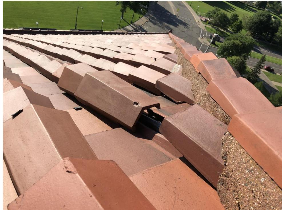
Overall Age of Roofing System, Areas of Cracked Terra Cotta Tile, Missing Nails, Leaks in Various Locations, Roof Trusses and Joists Structurally Sound
