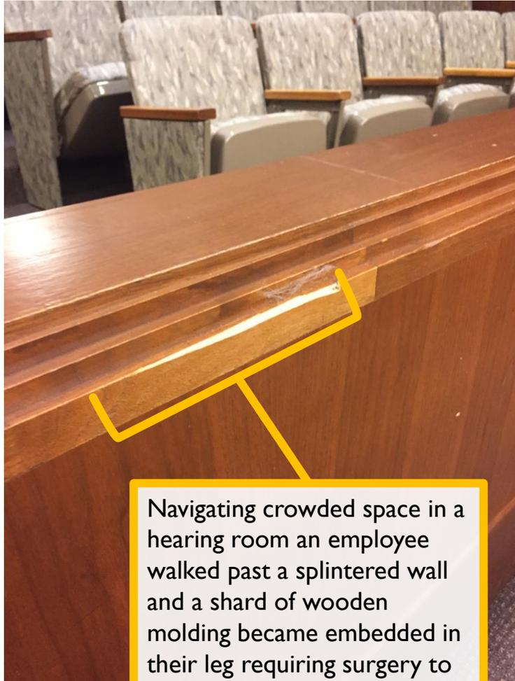
Navigating crowded space in a hearing room an employee walked past a splintered wall and a shard of wooden molding became embedded in their leg requiring surgery to remove.
