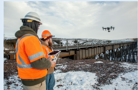
Rail employees use a drone to inspect a bridge.
