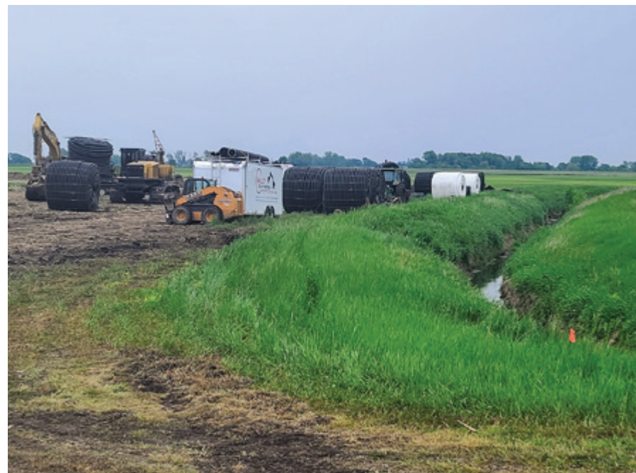
A History of Land Management Clay drain tile pipes were once laid by hand as shown in this historic photo (left) of early Minnesota farming. (Ayer, Harry Darius, circa 1910, Minnesota Historical Society) Modern equipment (right) like excavators and tile plows allows farmers to install perforated plastic piping quicker and easier.
