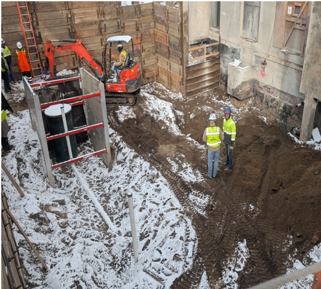
Loading Dock Excavation
