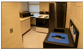
Small, outdated restrooms and break spaces
