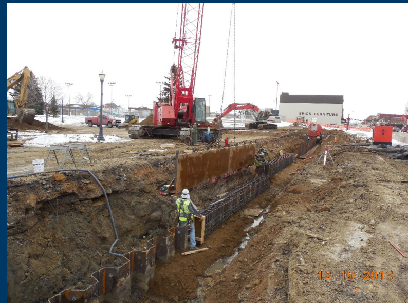
Flood Hazard Mitigation project in Austin, MN
