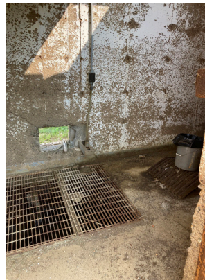
Aging bar screen with corrosion issues
