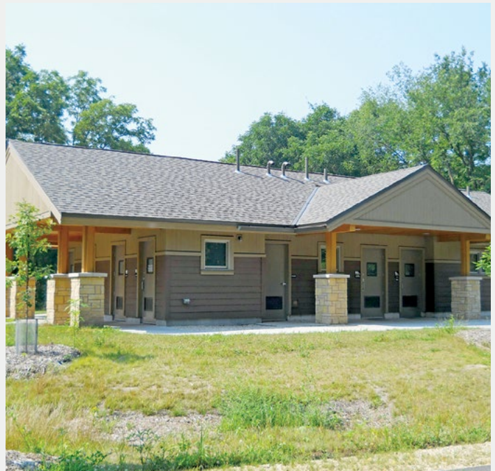
The replacement shower building, constructed in 2020 as part of a larger campground rehab project funded by a mix of Legacy and 2018 NRAP funding. The new building meets modern code, energy and water efficiency, and accessibility requirements, and also meets the expectations of park campers.
