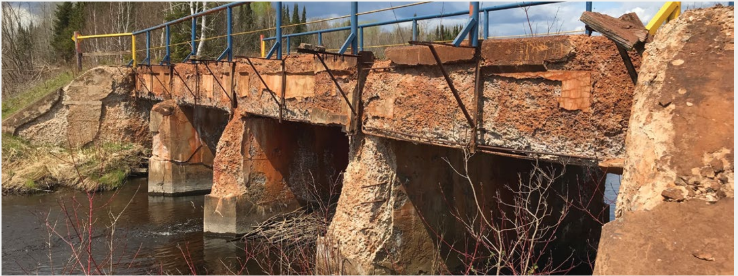
Above: Alborn-Pengilly Trail. This old railroad bridge shows complete failure of the concrete surfaces, exposing structural reinforcing steel to corrosion. This bridge must be completely replaced; it is not repairable.
