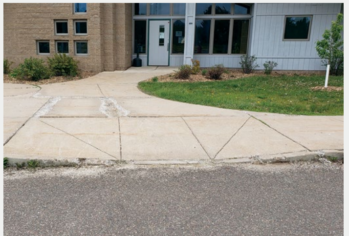
Aitkin office sidewalk.
