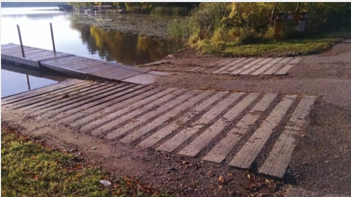
Before: Lake Alexander west access prior to rehabilitation.
