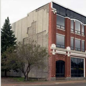
Ford Building Site $3.626 million GO
