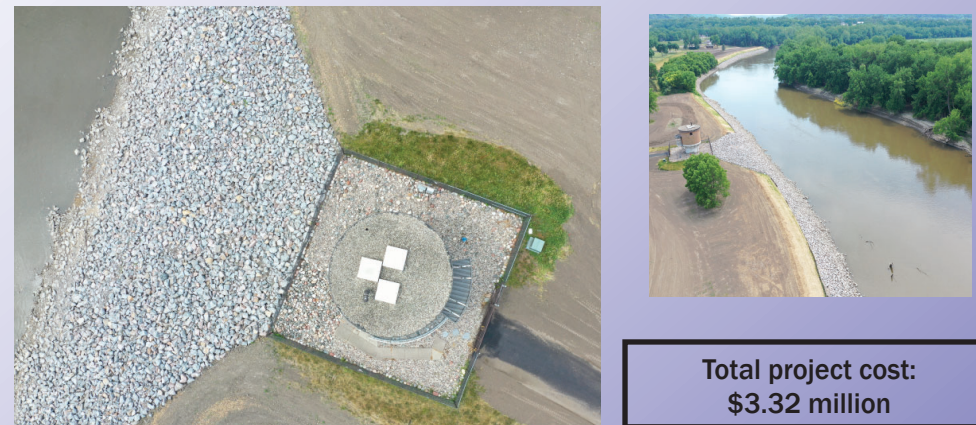
A view of Well 15 after riverbank stabilization.
