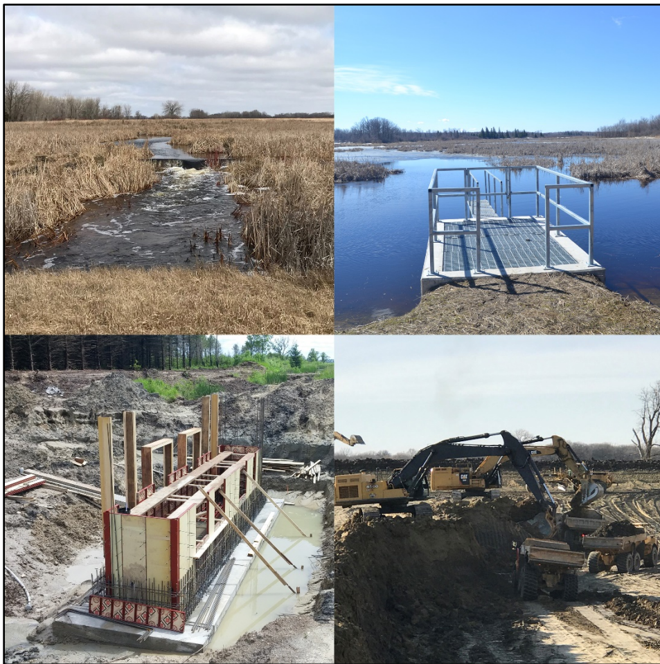
Constructed by local WDs in the RRB, FDR projects provide many societal benefits. Upper left: Lake Ida flood control weir dam in the Wild Rice WD. Upper right: water control structure at Little Pine Wildlife Management Area in Red Lake WD; lower left: dam structure forms at Roseau River Wildlife Management Area in Roseau River WD; lower right: Black Lake impoundment construction in the Red Lake WD.
