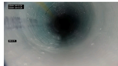
Post-liner installation
