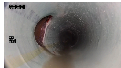
Post-liner installation
