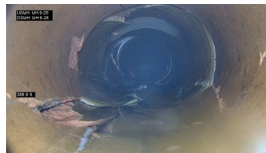
Pre-liner installation
