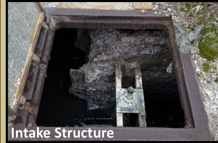
Erosion at WWTP
