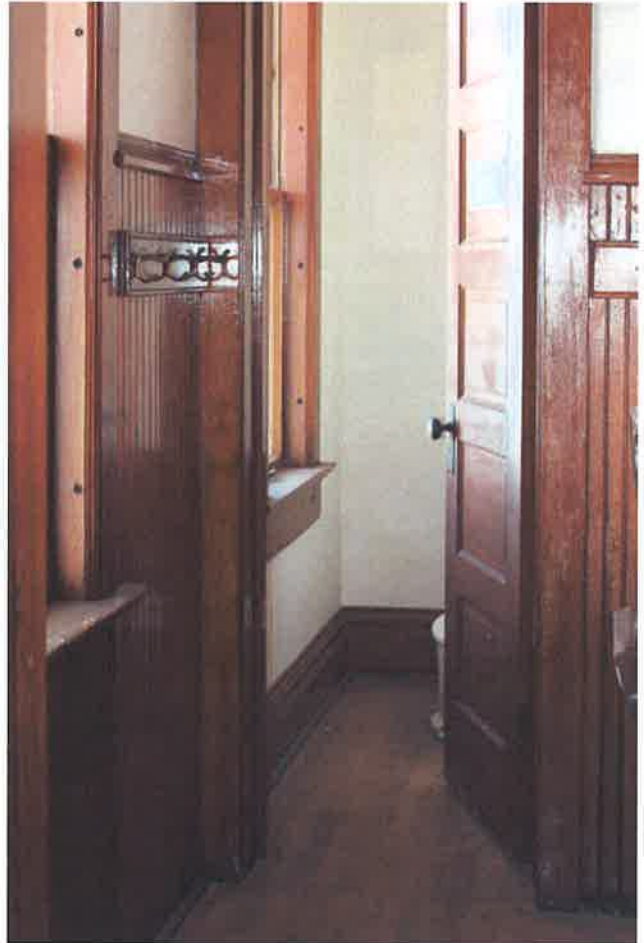
Original 1912 Toilet Facilities (not functional; not handicap accessible)
