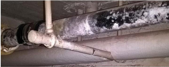
Domestic cold water line leaks and is causing corrosion and wear on the piping and surrounding areas.
