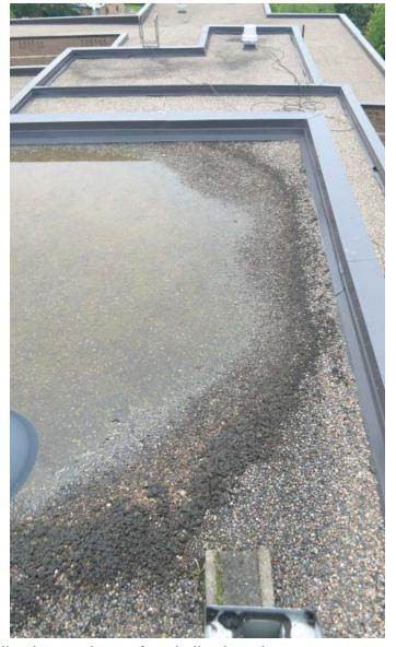
Roof is not sloped correctly in places. Moisture is collecting on the roof and allowing plants to grow. Replacement is needed for all but the western portion.
