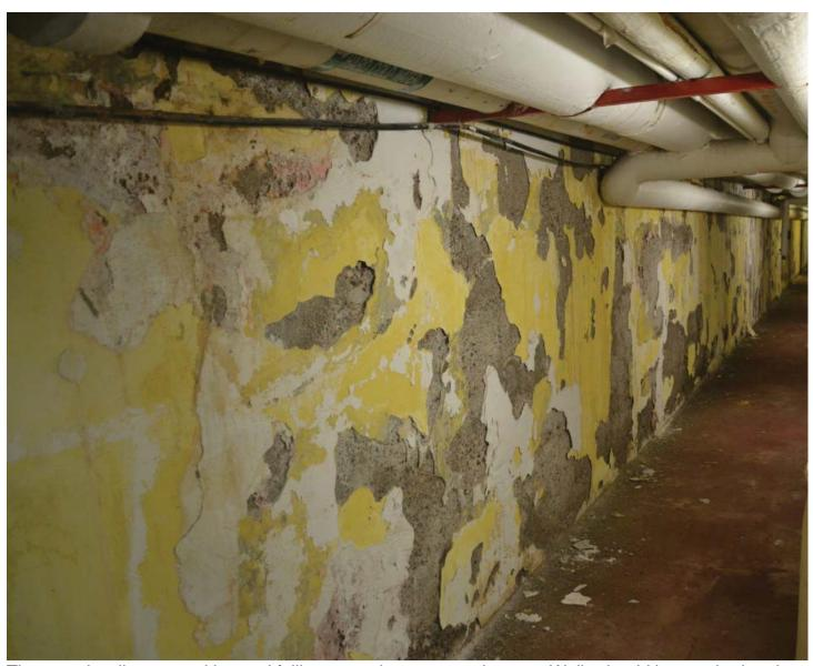
The tunnel walls are cracking and falling apart due to water damage. Walls should be repaired and resealed in order to prevent further damage.
