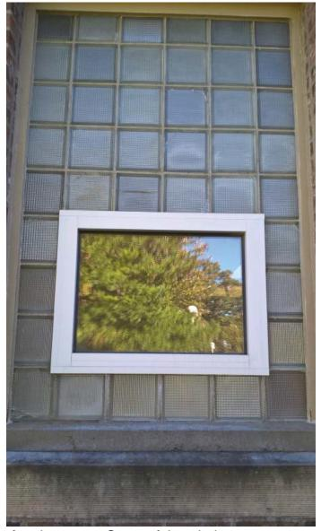
Glass block is cracked in many areas and is in need of replacement. Some of the windows are leaking to the interior.
