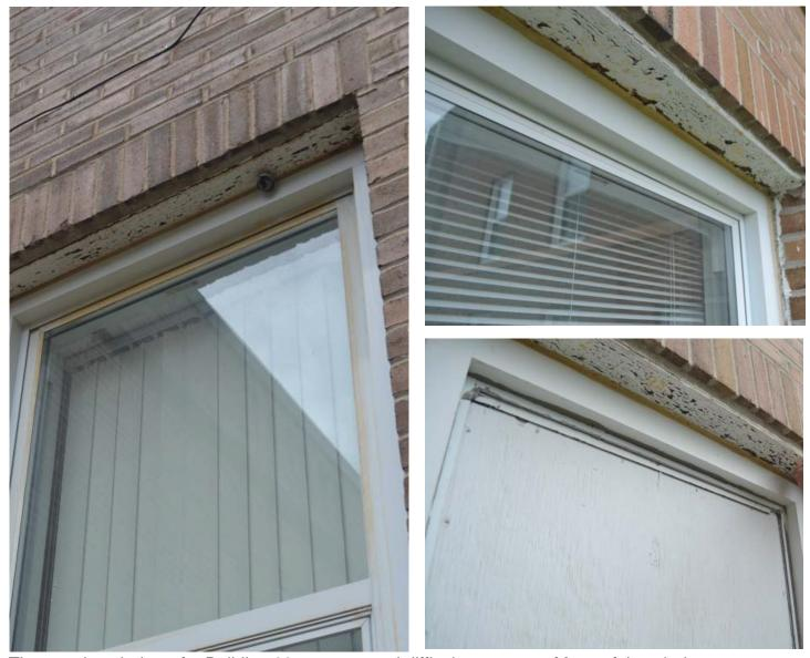
The exterior windows for Building 23 are worn and difficult to operate. Many of the windows are unable to be opened and closed.
