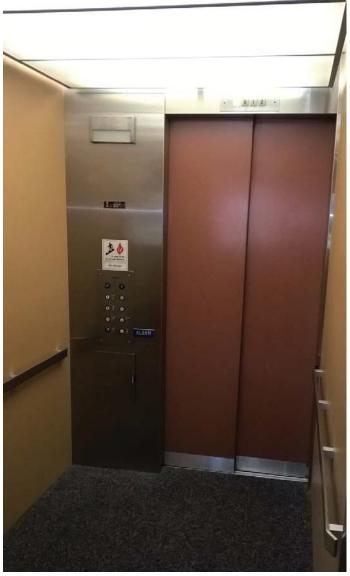
Elevator hydraulics are aged and obsolete. Rated as Poor based on age and condition and should be replaced.
