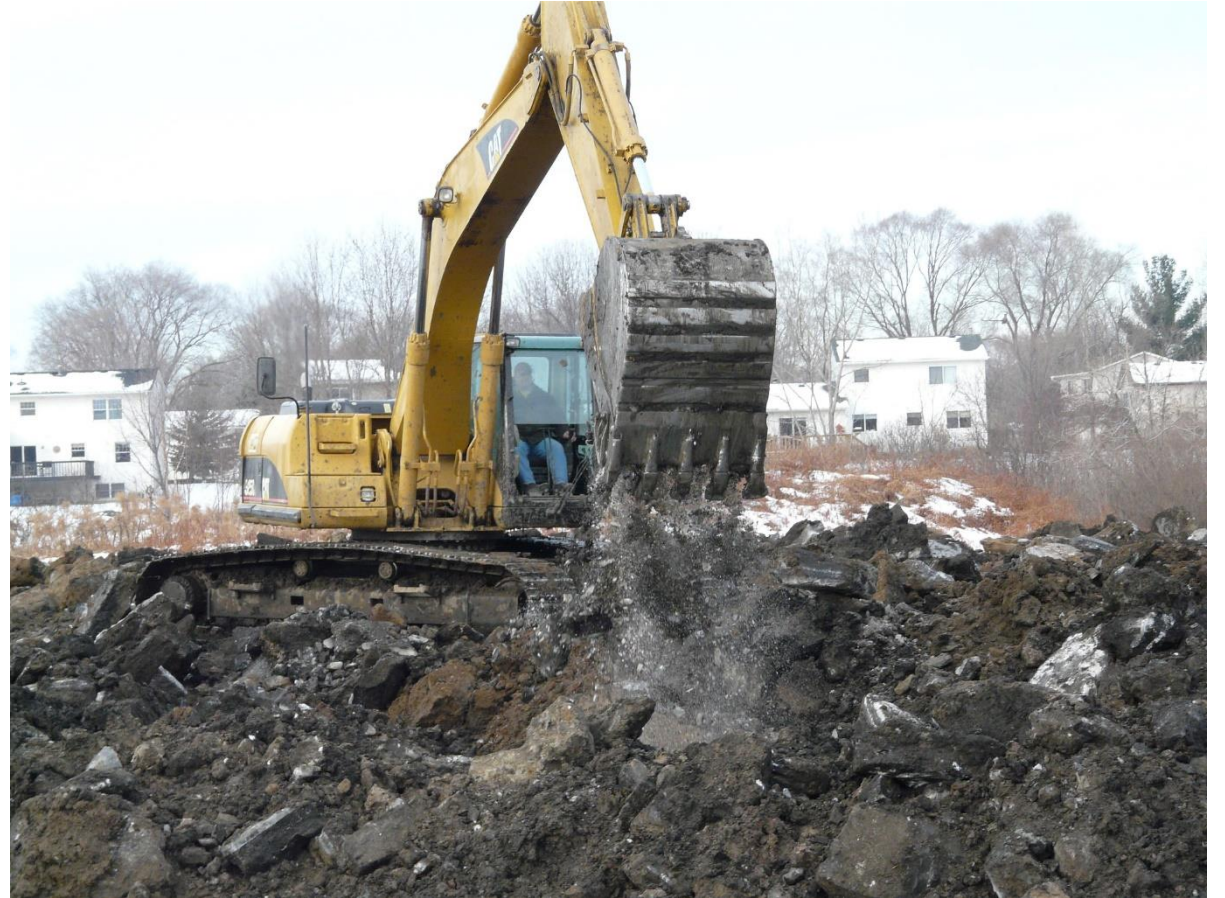
Removing sediment from a stormwater pond in White Bear Lake.
