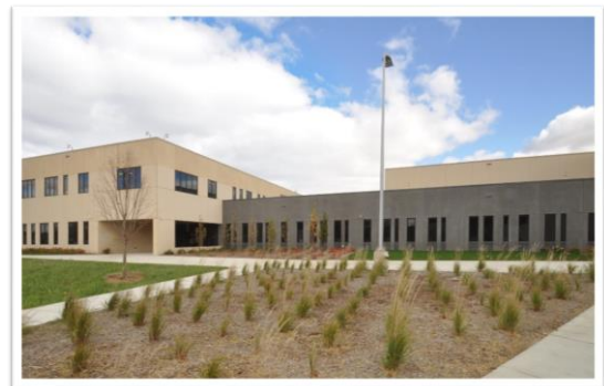
Minnesota Security Hospital, Phase 1
