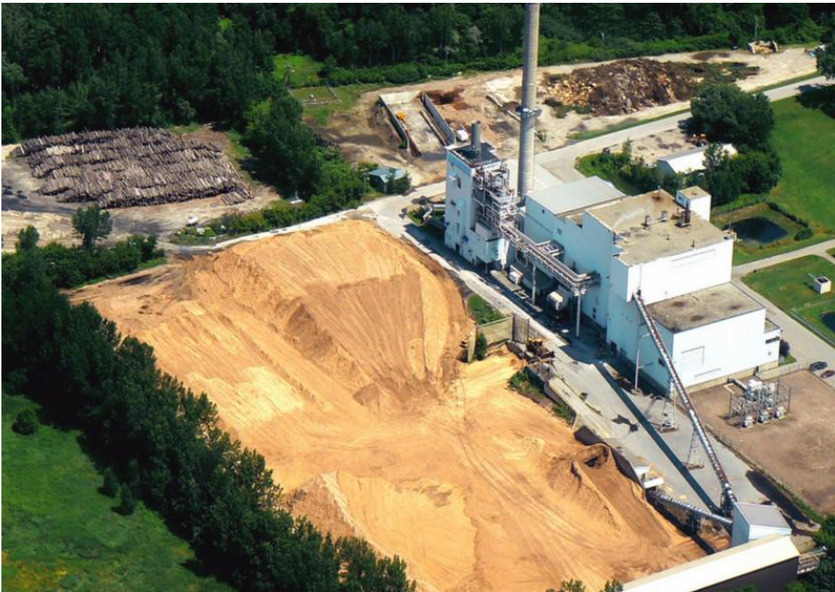
McNeil biomass plant in Burlington, Vermont: Piles of whole logs awaiting chipping. [photo: Chris Matera, Massachusetts Forest Watch]
