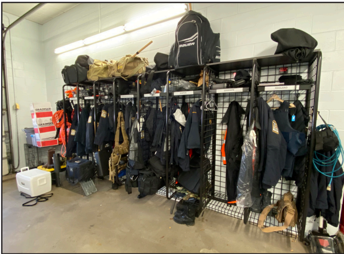
Locker room facilities are at maximum capacity, and do not provide officers with the space needed to sufficiently store personal effects. Additionally, equipment lockers are often shared as there is not space to add more.
