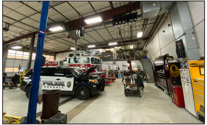
Exhaust fumes, caused by diesel particulate matter and carbon monoxide, exist in the building from the indoor mechanics' bay and indoor vehicle storage.
