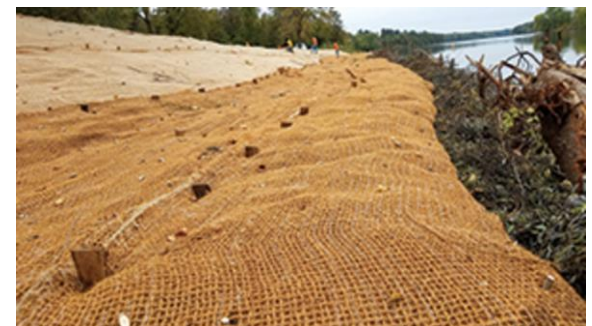
Natural fiber erosion control blanket.
