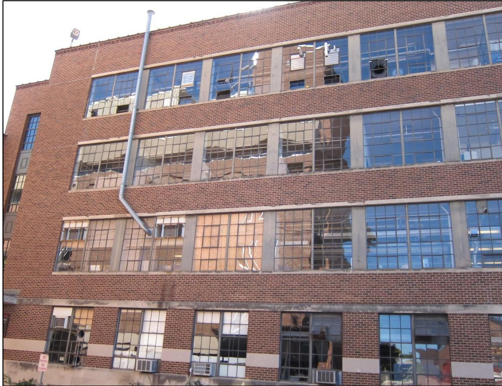
Left: Mechanical Engineering Building; improvised HVAC piping, window A/C units, and makeshift window coverings Right: Typical lab interior pre-renovation
