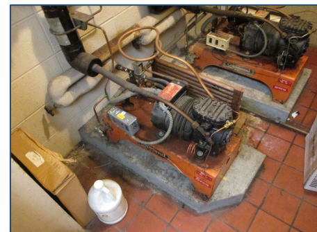
Right: TC - McNeal roof standing water (top); Food Sci. Nutrition - aged refrig. compressors (bottom)
