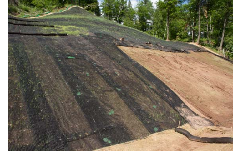
Turf Reinforcement Mat, intended for long term placement
