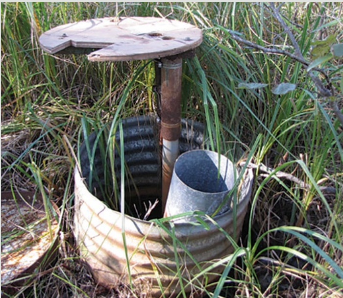
Monitoring well on state forest land in Aitkin County in poor condition.
