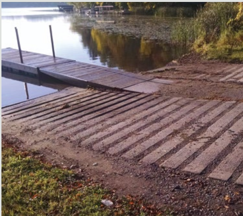
Lake Alexander west access prior to rehabilitation.
