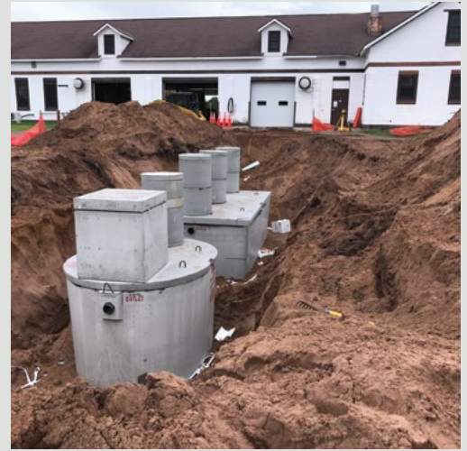
Septic replacement under construction.
