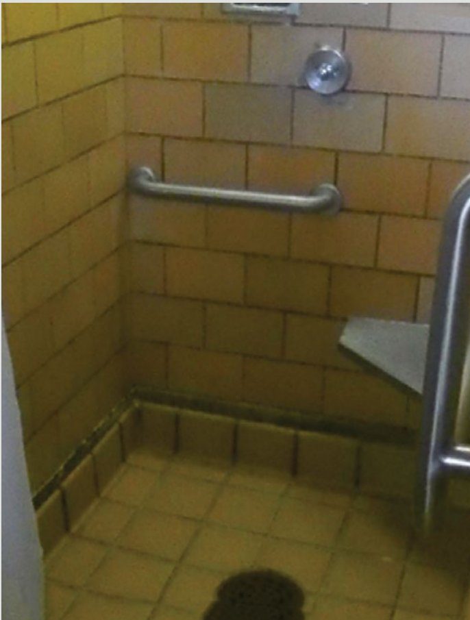
St. Croix State Park Riverview campground shower building.
