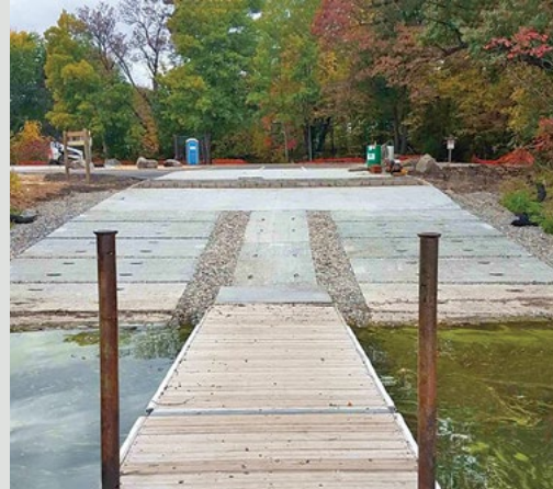
Lake Alexander west rehabilitated access.
