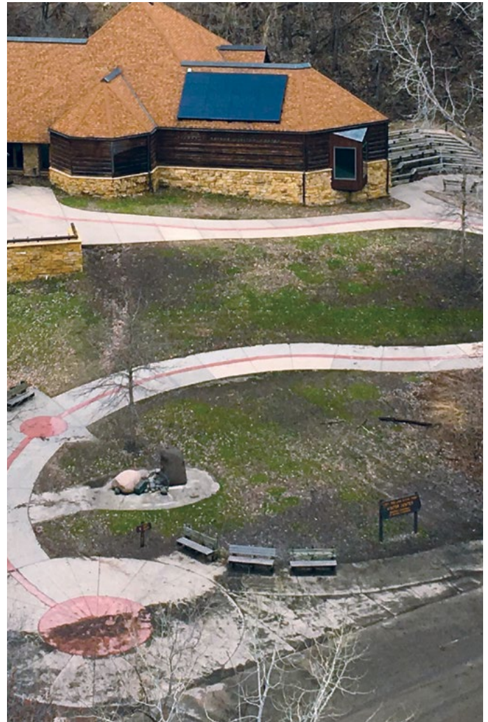
Aerial view of walkway to Fort Snelling State Park building entrance. The sidewalk exceeds ADA grade standards.
