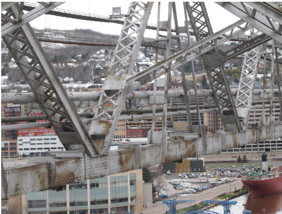
Corrosion, Steel Section Loss and the need for Repairs and New Protective Paint Coating System to the Overhead Truss
