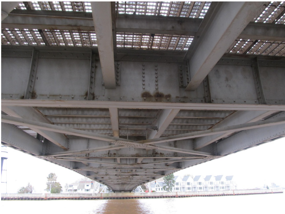
Additional View- Underside Lift Span Truss Protective Paint System Failure
