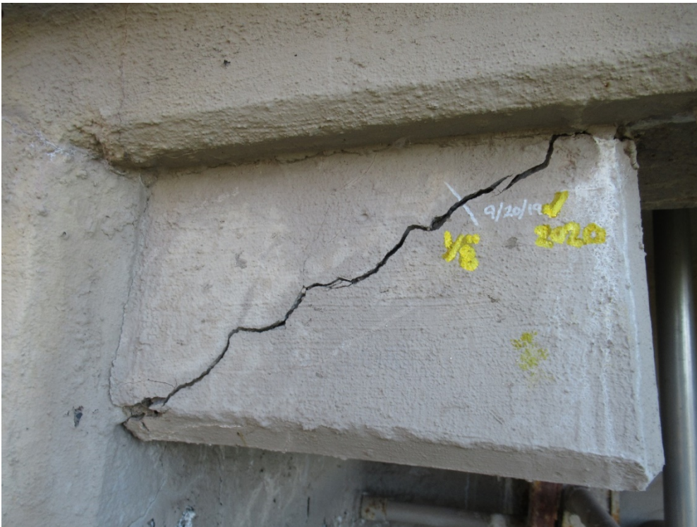
Cracking in Northwest Corner Concrete Sidewalk Support Beam
