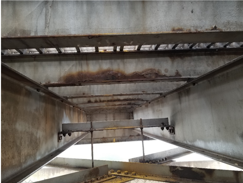
Rust and Corrosion from Road Salts is Necessitating Steel Repairs and New Protective Paint System to the Lower Regions of the Bridges Lift Span Truss
