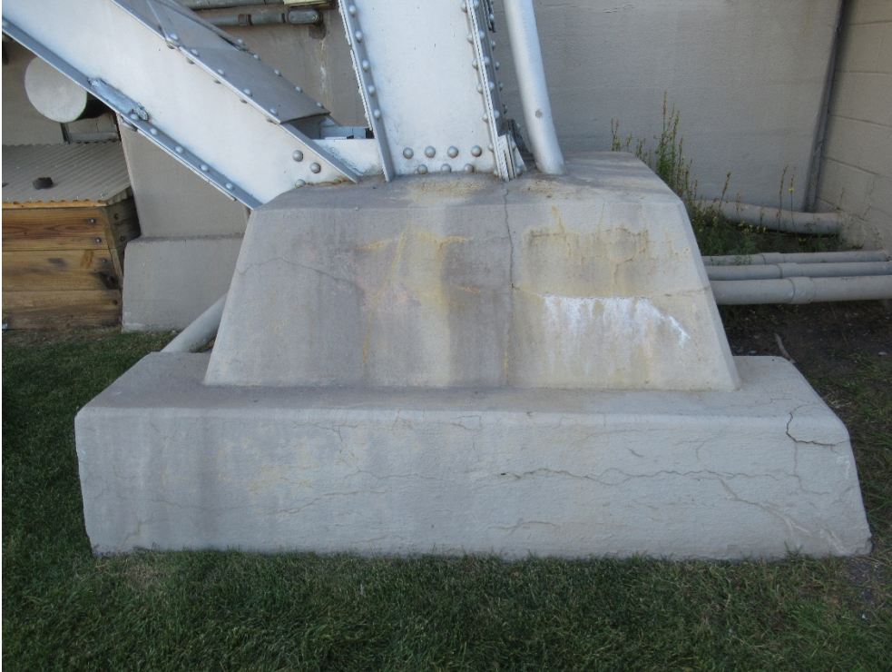
Cracking and Delaminations in Southwest Corner Tower Leg Concrete Footing
