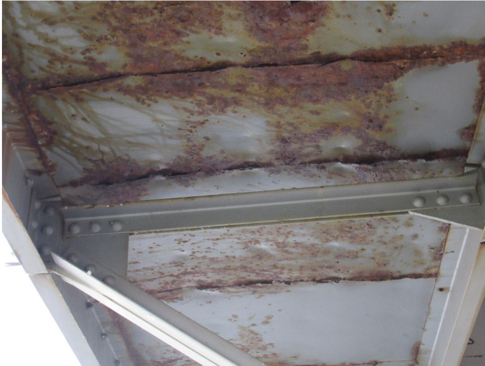
Steel Section Loss and Corrosion to Underside of Supported sidewalk on Lift Span
