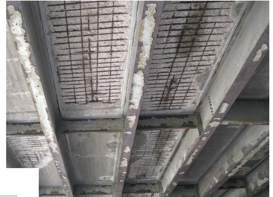
Maryland Ave. over I-35E (before reconstruction)
