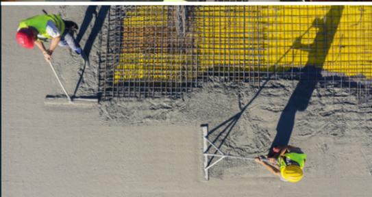
3M™ Natural Pozzolans, a SCM (supplementary cementitious material) used in the making of concrete, helps reduce CO<sub>2</sub> emissions as a partial replacement of cement in concrete.<sup>2</sup> It's estimated that each ton of SCM used to displace cement reduces CO<sub>2</sub> emissions by 0.75 tons.<sup>3</sup>
