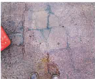
Leaking Water Service in Tracy, MN
