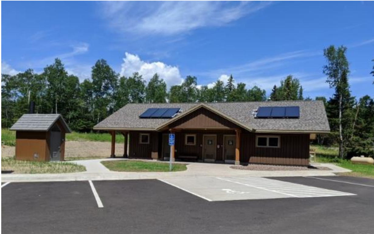
Temperance River State Park – New Shower Building Park users expect clean, modern, family-friendly and climate-friendly facilities.
