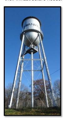
The City's only water tower was constructed in 1931. Now over 90 years old this tower is undersized, provides substandard pressure to parts of the community and has aged far beyond the point of rehabilitation. In February 2020, the MN Department of Health issued a letter to the City that required *Correction of Significant Deficiencies* which required costly emergency repairs to keep the reservoir in service. Despite the emergency repairs, this reservoir is in desperate need of replacement.
