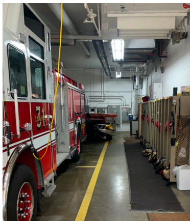
Figure 1: Firefighters must dress adjacent to moving vehicles.
