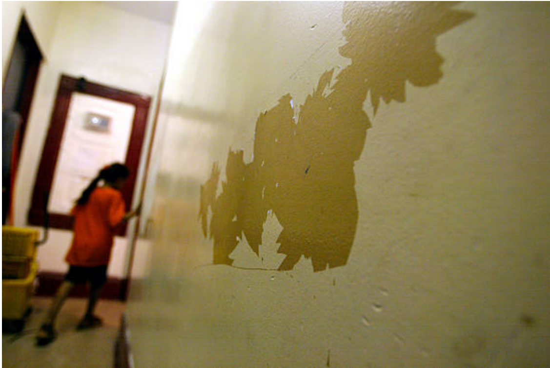
Children walk past peeling lead paint. Children ingest lead paint and lead paint dust, resulting in lead poisoning, which causes irreversible brain and central nervous system damage. Photo by Spencer Platt/Getty Images.
