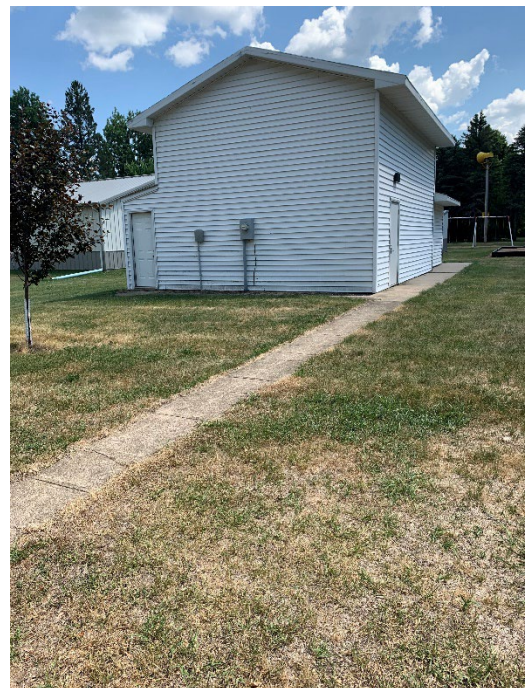
Figure 1 Filter is housed in this building
